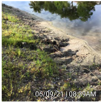
2. Figure 2 - Minor Rilling and washout previously stabilized with riprap that has been washed out
