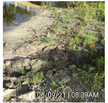
2. Figure 2 - Minor Rilling and washout previously stabilized with riprap that has been washed out
