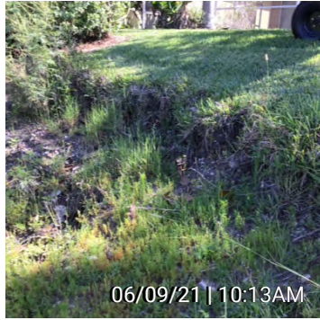
18. Figure 18 - Washout, extend downspout drain to lake
