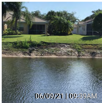
12. Figure 12 - Deep Rills from Runoff
