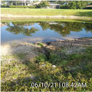
62. Figure 62 - Washouts throughout bank
