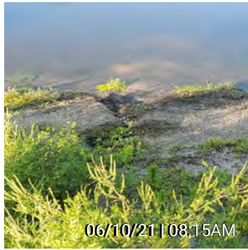
57. Figure 57 - Washout (Recurring)
