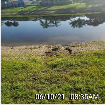
62. Figure 62 - Washouts throughout bank
