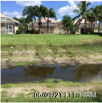
28. Figure 28 - Minor Washouts at Lake Bank
