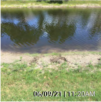
28. Figure 28 - Minor Washouts at Lake Bank
