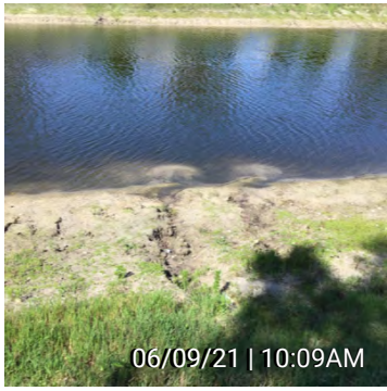
17. Figure 17 - Drop greater than 9" with washout
