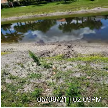
46. Figure 46 - Pool overflow causing washout
