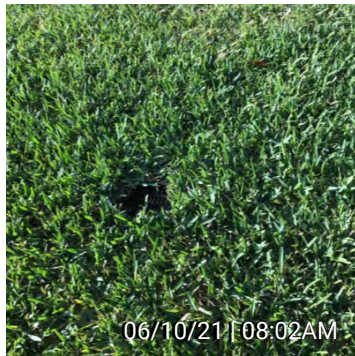
54. Figure 54 - Washout from bubble up Dan DiVincenzo | 07/08/21 | 03:38PM
