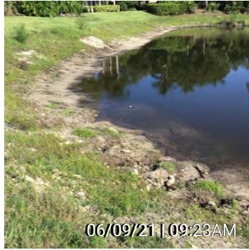
10. Figure 10 - Rilling from downspout drain (Recurring)
