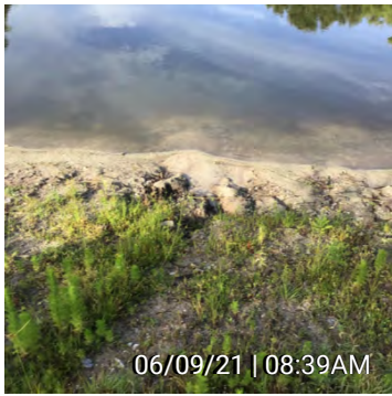
2. Figure 2 - Minor Rilling and washout previously stabilized with riprap that has been washed out
