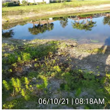
57. Figure 57 - Washout (Recurring)
