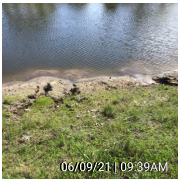
12. Figure 12 - Deep Rills from Runoff
