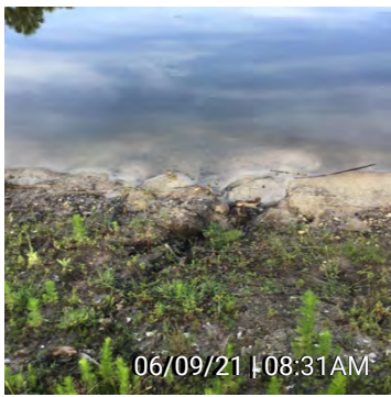
2. Figure 2 - Minor Rilling and washout previously stabilized with riprap that has been washed out
