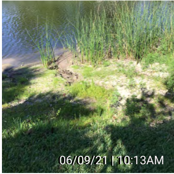
18. Figure 18 - Washout, extend downspout drain to lake
