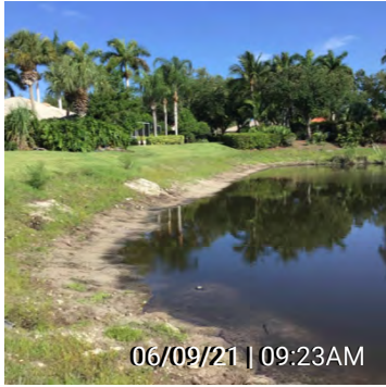
10. Figure 10 - Rilling from downspout drain (Recurring)
