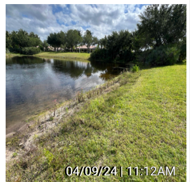
15. Lake 26 washout on the South side of lake/ stabilized over time. Noticed 1 aerator functioning in lake. Dalton Lehnhard | 04/11/24 | 03:34PM
